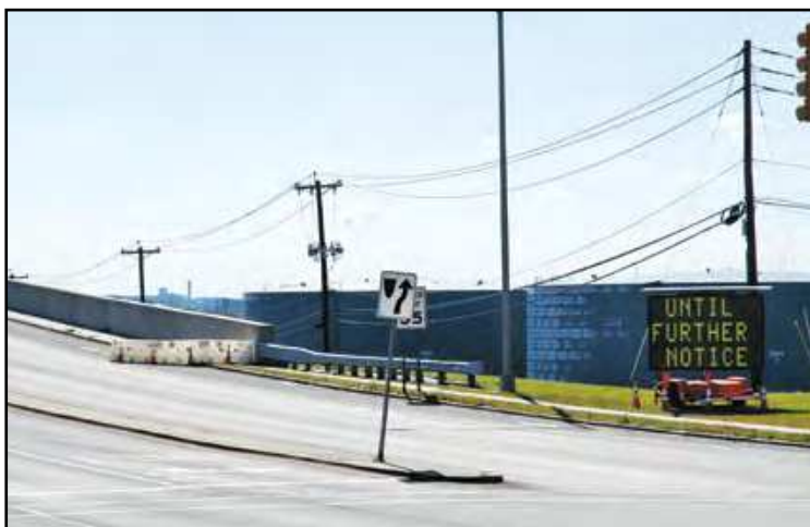
The walkway/bike path is blocked off at the Victory Bridge until further notice.
