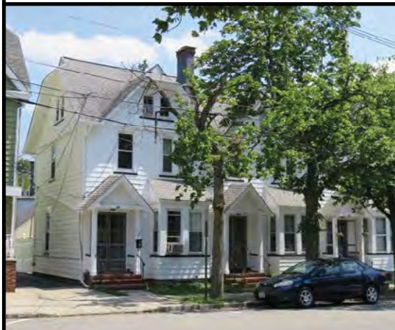
PERTH AMBOY - Unique 4 Family in the great Perth Amboy Water Front, all separated utilities including Water & sewer, only 3 water meters 208 apartment tenants splits water & sewer. Insurance is $2,856, perfect condition many upgrades a "must see." $539,900
