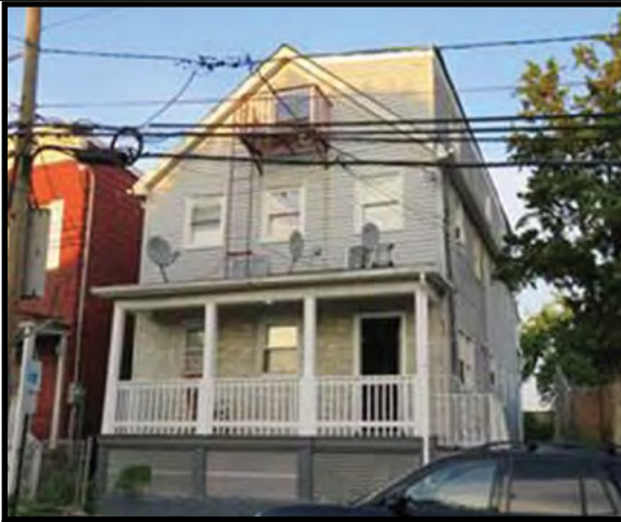
PERTH AMBOY - This is a fully rented 3 fam., separated utilities, close to most major public transportation and schools. Buyer is resp. for C/O and all repairs. $269,900
