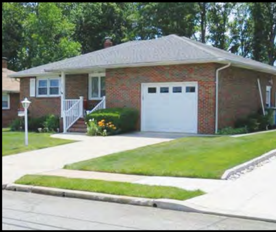
PERTH AMBOY - Superb custom built all Brick Ranch 3 bedroom, New windows & newer roof, single owner that took good care over the years, all hardwood floors, large basement, garage. Built in 1967. A "must see" and much more! You will love this home's location!! $264,800
