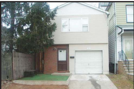
PERTH AMBOY - Beautiful home, needs a little TLC. Sold "as is". Buyer is resp. for all inspection and repairs. Nice Area. Close to train, bank, church and stores. $182,000
