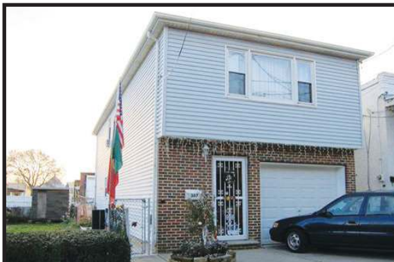
PERTH AMBOY - A must see this well maintained, large 3 bedrooms, 2 full bath, big house. Subject to subdivision. $219,900
