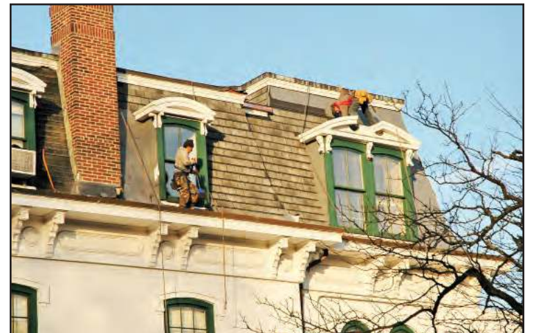
Repairs are being made to the Roof and Cupola at Perth Amboy City Hall photo by Paul W. Wang
