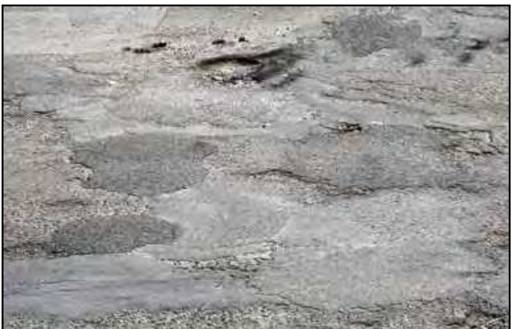
Portion of Stockton Street
