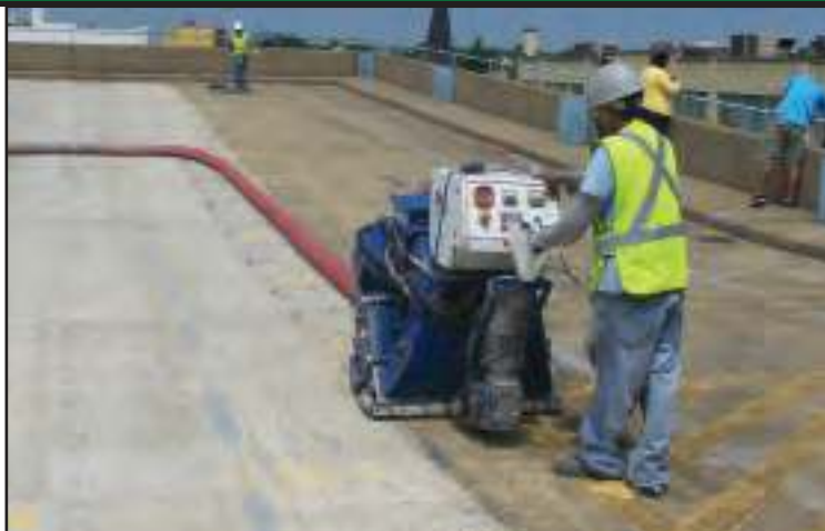
The renovations of the top floor of the parking deck gets started.
