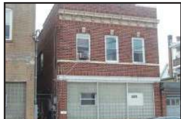
PERTH AMBOY - Excellent condition. Good investment. Roof 2 yrs old. Sold "as is." No questions asked. Property is in very good, "move-in" condition. $199,000
