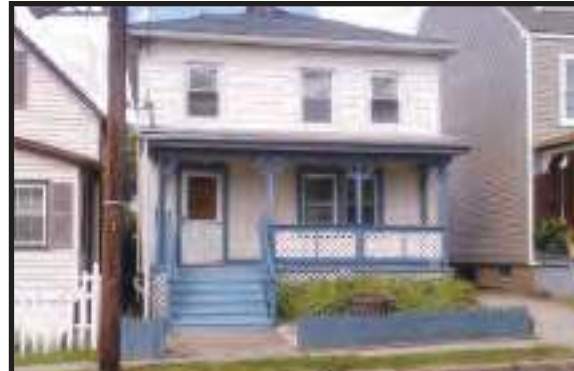
PERTH AMBOY - Nice size family home, offers 3 spacious bedrms, 2 full baths, master has a nursery/office. New roof, new windows & Pergo flrs installed throughout. Open flr. plan 1st level, tons of windows, so light & airy. Owners bonus full tank of oil (1.5 winters) . . . WOW! Estate Sale. Benign sold "AS IS" & C/O buyers resp. $149,900
