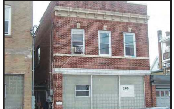
PERTH AMBOY - Excellent condition. Good investment. Roof 2 yrs old. Sold "as is" No questions asked. Property is in very good "move-in" condition. $185,000
