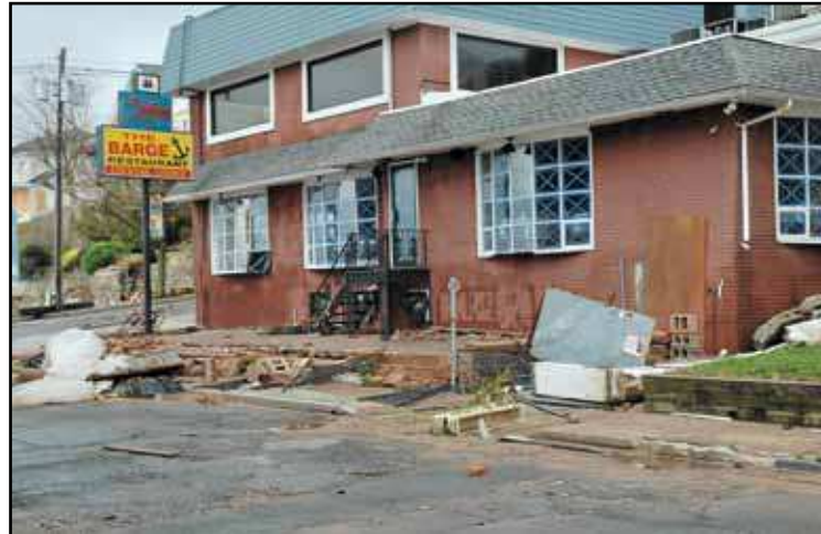
Damage to the Barge
