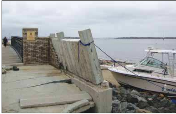
The wall was knocked loose
