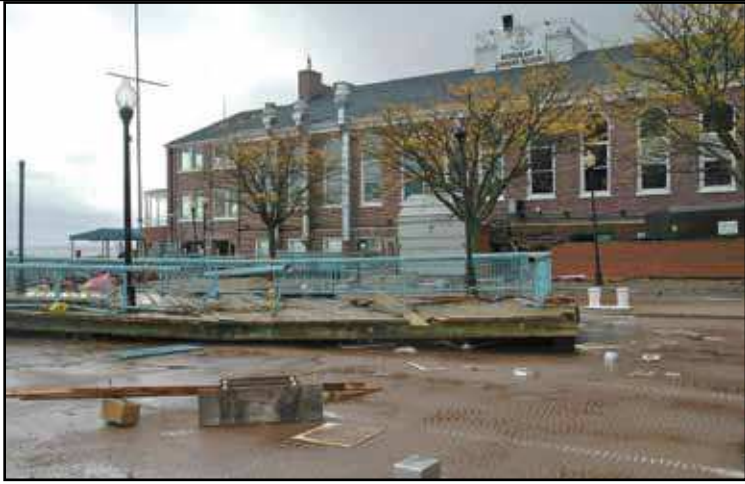
Outside the Armory
