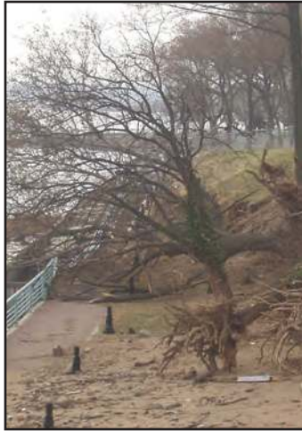
PERTH AMBOY - Trees uprooted in the Waterfront. Walkway damaged. *Photo by Joe Bayona
