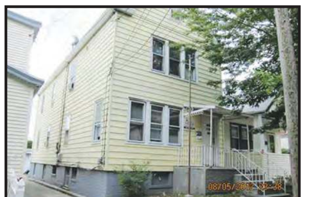
PERTH AMBOY - Great potential. Close to public transportation and all major hwy's. Buyer is resp. for C/O, Termite Cert. and all repairs. This is being sold strictly in "AS IS" condition. Only CASH, or FHA 203K. $159,000
