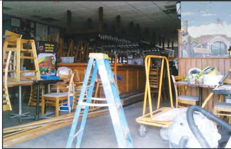
In Perth Amboy, the Barge is making great progress
