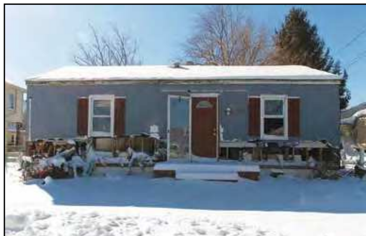
SOUTH AMBOY - Recent photos of houses devastated by Hurricane Sandy *Photos by Aaron Beers
