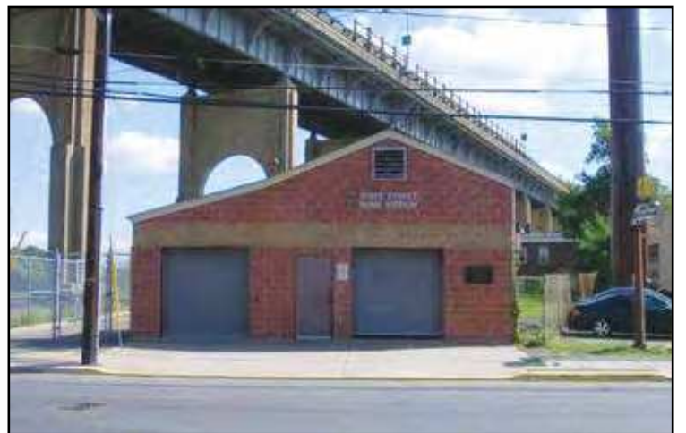
Perth Amboy Pumping Station at 800 State St.
