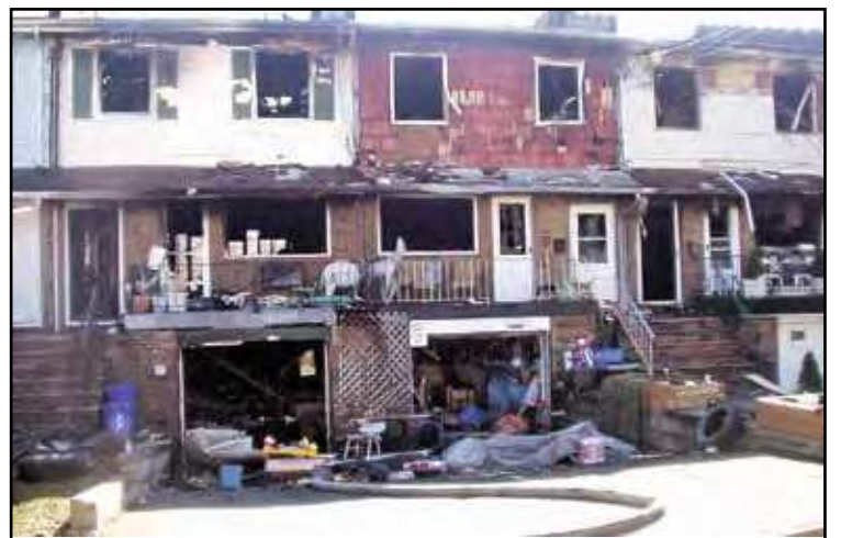
Damage due to the intensity of the fire
