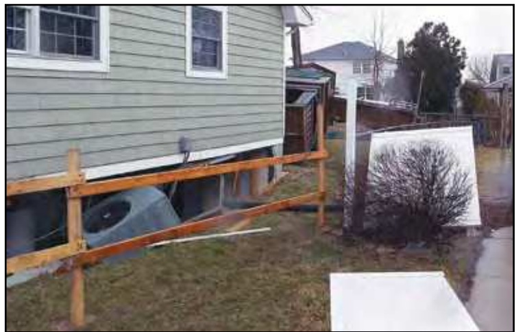
Equipment underneath the foundation
