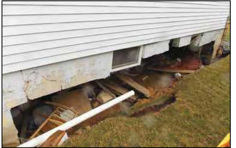
Debris underneath the foundation
