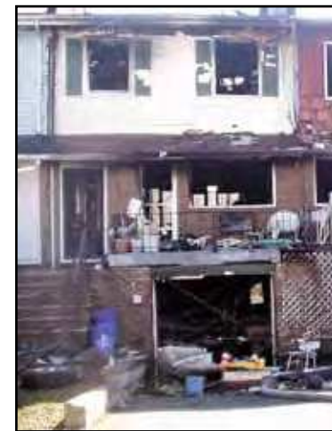
Rear of Fire at West Side Avenue
