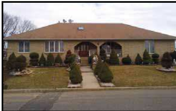
SAYREVILLE - Custom built home only 21 yrs. old. Too many upgrades to list. Home has over 4900 sq. ft. of living space. Huge lot, vaulted ceiling with skylight in foyer. Italian ceramic flr throughout fyr, din, kit, breakfast area, bsmt & all hallways. Hdwd in liv, fam & all 3 bdms. 2 C/A (1 for liv+ 1 for slpng). $449,900
