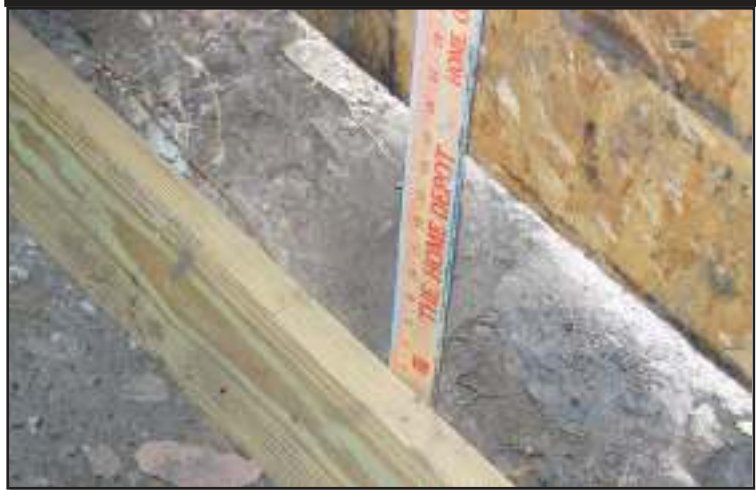
Tom Ward shows damage to his garage
