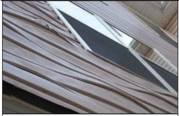
Siding buckling
