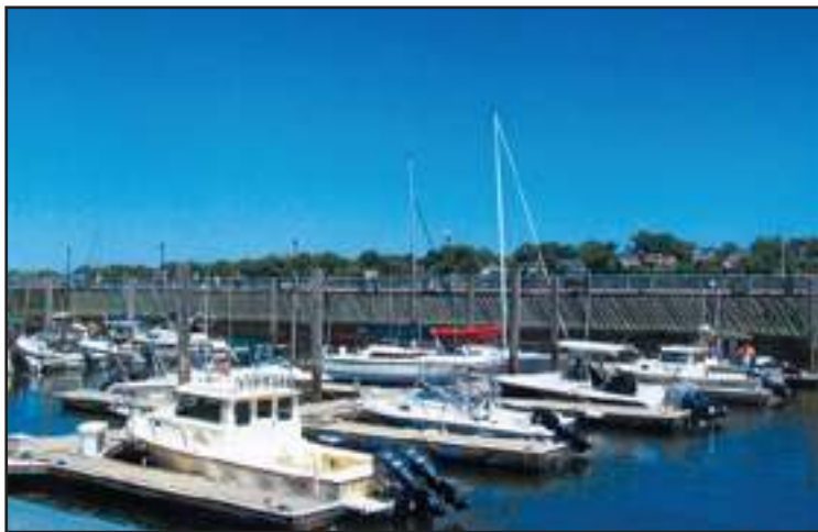
Photos show the Perth Amboy Waterfront that was destroyed by Hurricane Sandy shows signs of life every month *Photos by Carolyn Maxwell
