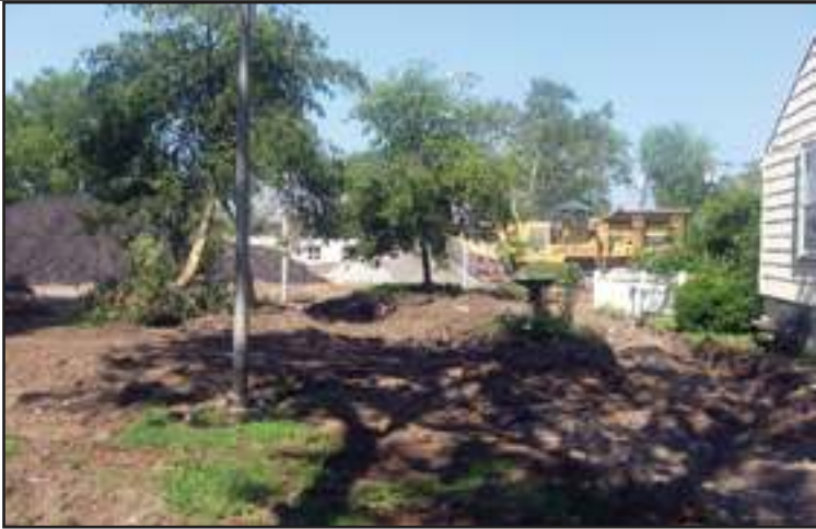
Working on the Tennis Courts
