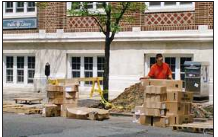
PERTH AMBOY - Sidewalks are dug out in front of the Perth Amboy Public Library on Jefferson Street. This is part of the improvements needed before the main level can be reopened to the public.
