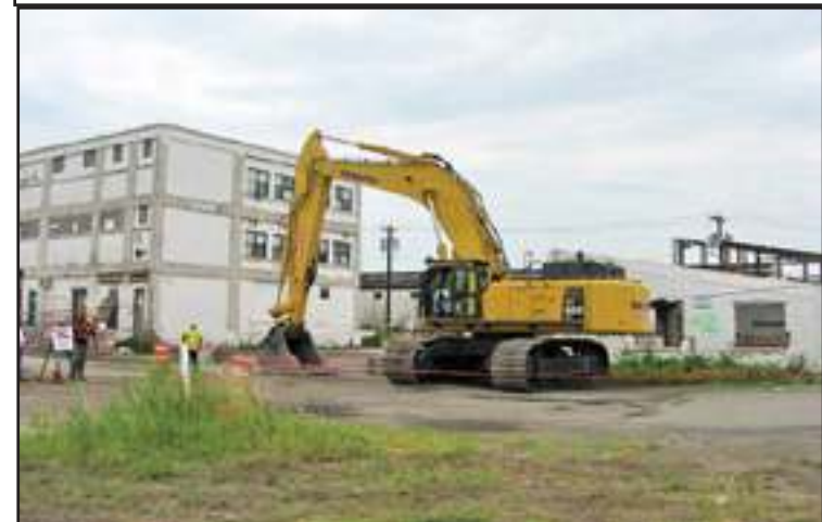
The first building just before it is demolished
