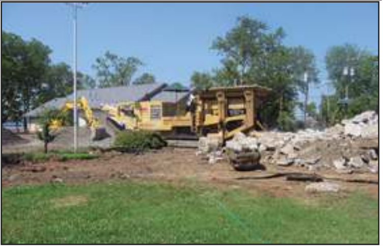
Working on the Tennis Courts
