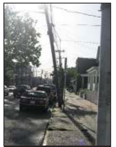
PERTH AMBOY - Market Street (by Madison Avenue). A Telephone Pole leans into the street. *Photo by Katherine Massopust
