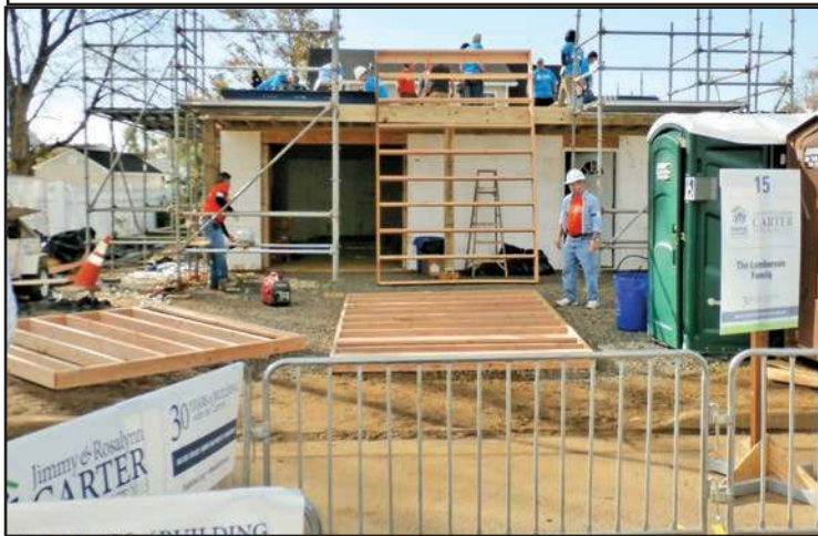
The House under construction
