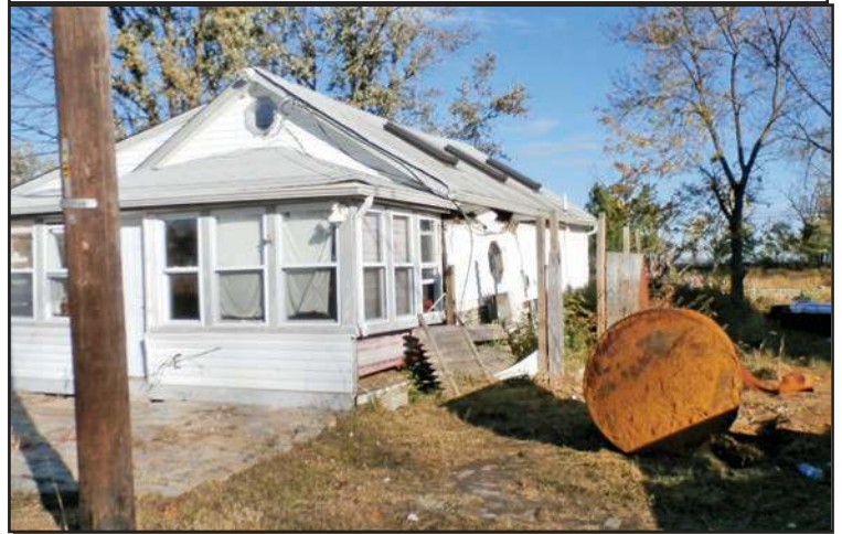
One of the houses in Union Beach damaged by Sandy
