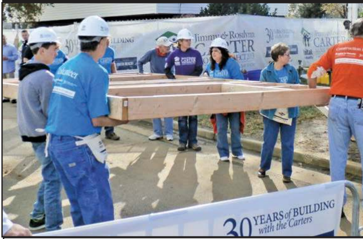
Volunteers carry part of the frame of the House they were building
