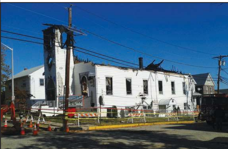
PERTH AMBOY - SS. Cyril & Methodius National Catholic Church suffered extensive damage to the roof during a 3 alarm fire which occurred around 1 a.m. Monday, Oct. 28, 2013. The Church was 90 years old. *Photo by Katherine Massopust
