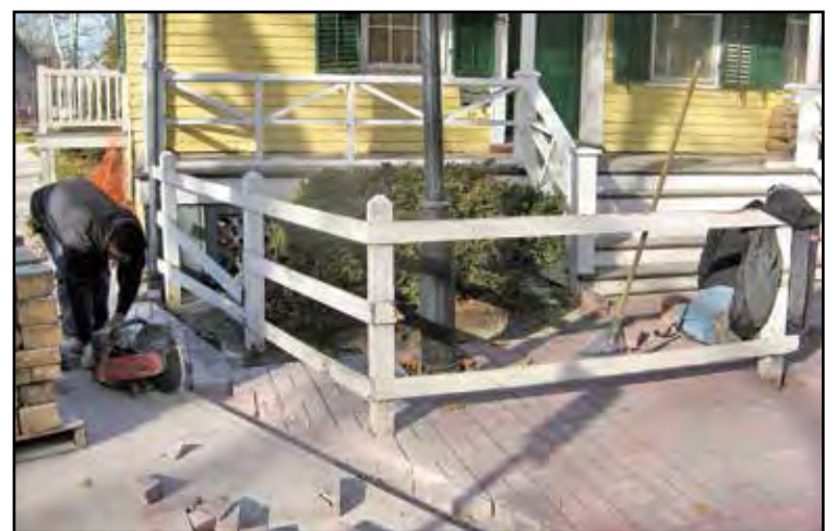
Workers laying the bricks at the Kearny Cottage
