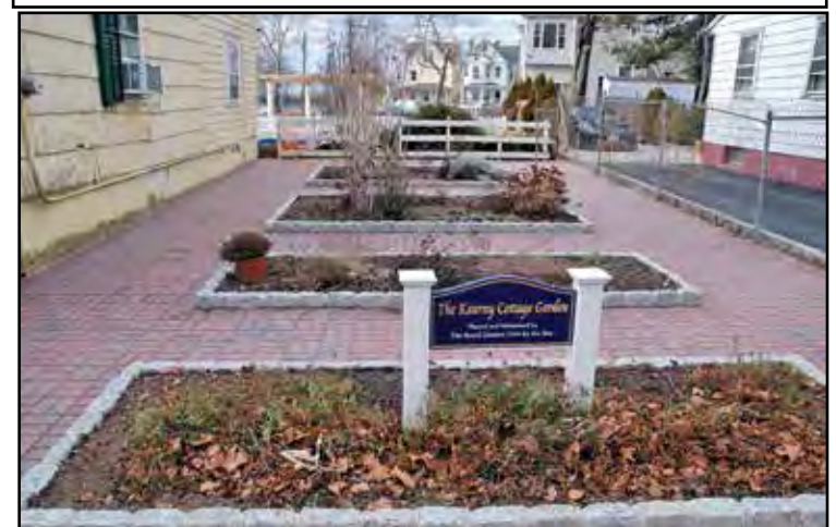
The completed brickwork
