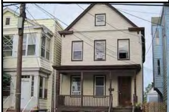
PERTH AMBOY - This Property is in the heart of Perth Amboy, great potential needs some TLC, is being sold in "As IS" condition. buyer is responsible C/O and repairs 203K or cash. $165,000
