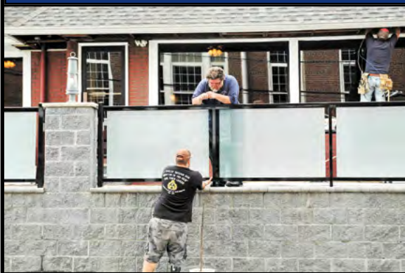
The Glass enclosure was installed by R&S Glass
