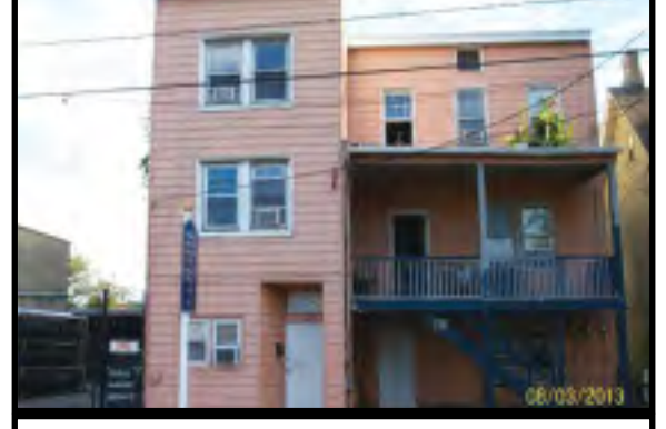
PERTH AMBOY - CALLING ALL INVESTOR. ACTUAL INCOME IS FROM LONT TIME TENANTS. LOT OF POTENTIAL. SHOW AND BRING OFFER, SELLER VERY MOTIVATED TO SALE. !!!!24 HOURS NOTICE!!!! BUYER RESPONSIBLE FOR ANY INSPECTION CERTIFICATE AND REPAIRS. $299,000
