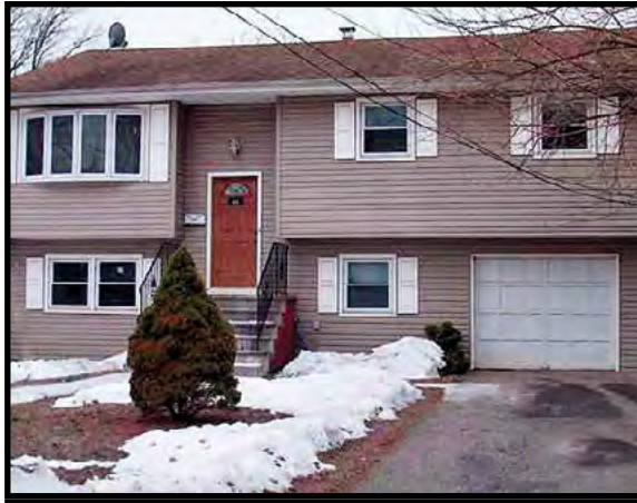
SEWAREN - VERY NICE MOTHER AND DAUGHTER. THIS IS A SHORT. HOUSE HAS DAMAGE FROM SANDY IN PROCESS OF RENOVATION. $209,900
