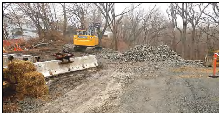
SOUTH AMBOY - Sinkhole due to Water Main Break *Photo by Joe Bayona
