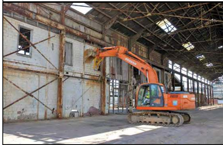
The Demolition Begins!
