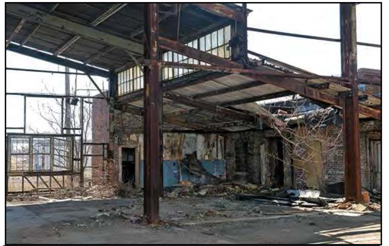
The last remains of AS&R. Photo taken 4/1/15 when demolition began. *Photos by Katherine Massopust
