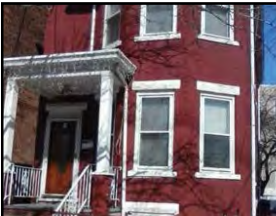
PERTH AMBOY - Nice house for large family. Buyer is responsible for C/O and any repairs. $189,000
