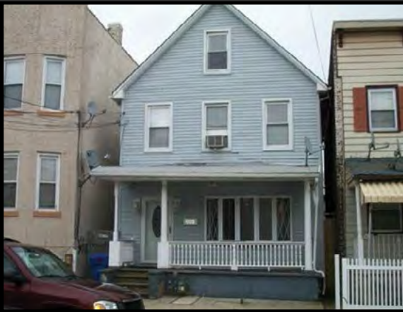
PERTH AMBOY - Nice 5 bedrooms and 4 bath house, Sold "As Is Condition". Buyer Resp. for C/O Inspection. $229,000
