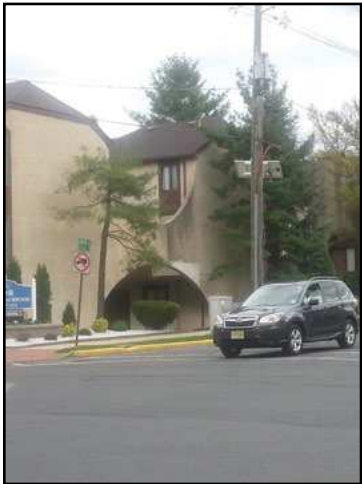
Both Photos above show Part of the 200 Block. It is located NE of City Hall on High Street with mixed use buildings, most which have their own parking garages or private lots.
