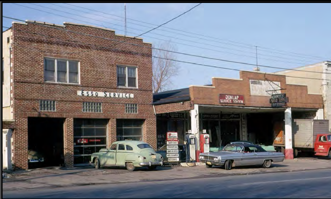
PERTH AMBOY - Dunlap Service Station and Garage, Circa early 1960's. Amboy Avenue across from Keene Street.
