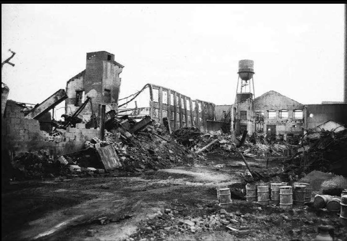
PERTH AMBOY - Cableworks Fire on High Street July 9, 1980. The Fire Burned for 9 Days. The fire was believed to be caused by a spark that was near cleaning solvents. Many Fire Departments were called to the scene.
