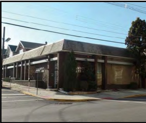
PERTH AMBOY - Great opportunity for Doctor office located across the street from RBMC, a well established medical facility. 2 separated furnace and hot water, 2 baths, storage space sprinkler system only downstairs. 3 parking spaces, 2000 sqft rented for $2,500 Mo to Mo. 3000 sqft Vacant. $500,000
