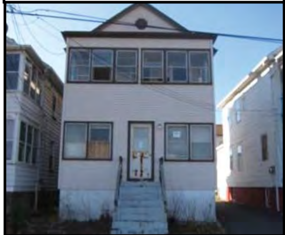
SOUTH RIVER - Great Potential. Handyman Special. Is Being Sold "as is." Buyer resp. for smoke cert., termite cert., and all repairs. $168,000
