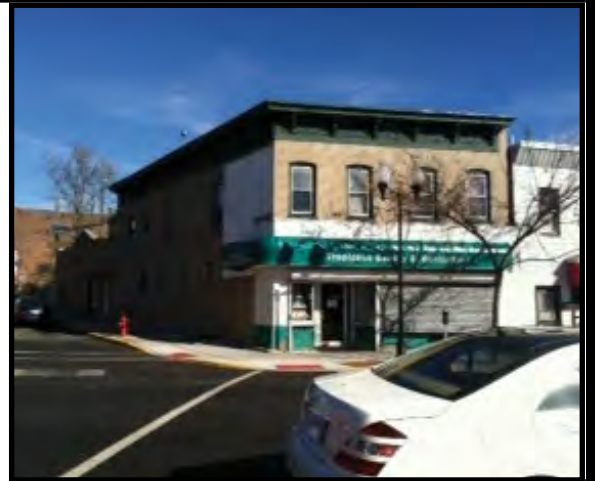
PERTH AMBOY - Great location, high visibility, office, warehouse or store. Space has been going under major renovation, roof, HVAC, windows, electrical, plumbing, floors, insulation, new drywall(wall/ceiling). Look at the new pictures attached for a better idea. $1,800/Mo Rent
