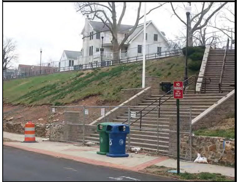
Another view from Front Street looking upwards. Work being done is supposed to shore up the wall and foundation to strengthen the structure of Bayview Park.
