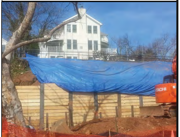
A tarp covering the newly built wall that will reinforce part of Bayview Park.
