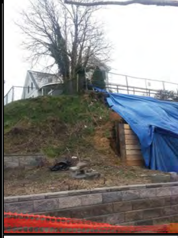
Photo taken from parking lot on Front Street, looking towards Bayview Park
