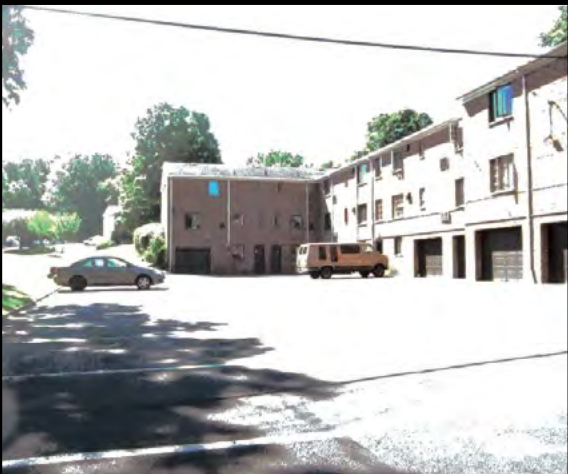
SPRINGFIELD - Being sold strictly in "AS IS" condition buyer is resp. for Smoke Cert., Termite Cert. and all repairs. $134,900
