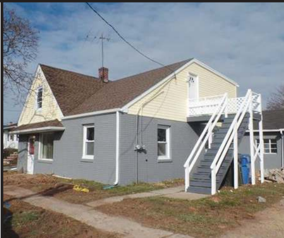
HOPELAWN - A truly move-in condition two family a must see. This property has the garage you have been dreaming of in this terrific location. it is in mint condition, very nice kitchens all painted and much more. $269,000
