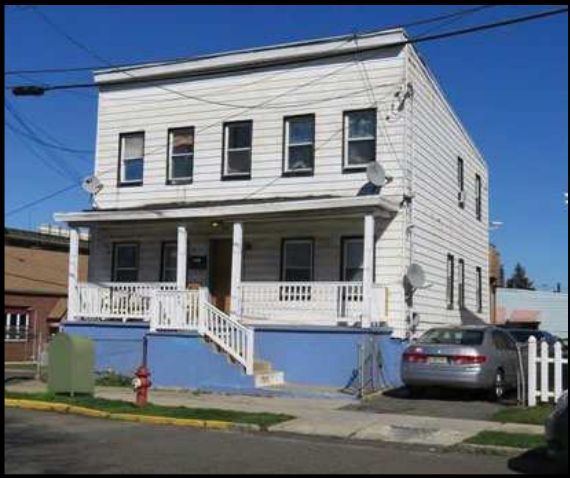
PERTH AMBOY - Great Investment needs some TLC 4 family in front and single family in rear. 4 units are rented for $800.00 each Mo to Mo. Owner pays water and heat. 5 electrical and gas meters. In-ground in use oil tank. $324,900
