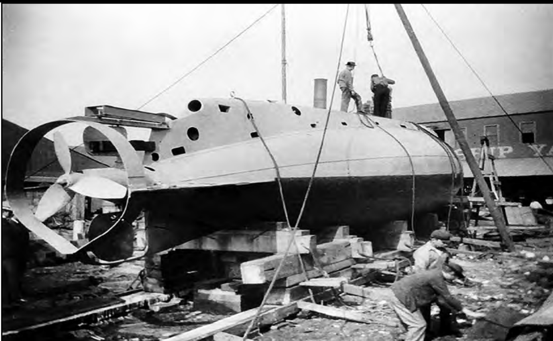
PERTH AMBOY - The Holland , the first U.S. Submarine in Dry Dock at the Schantz and Eckert Machine Works. The company built some of the machinery for the Holland .
