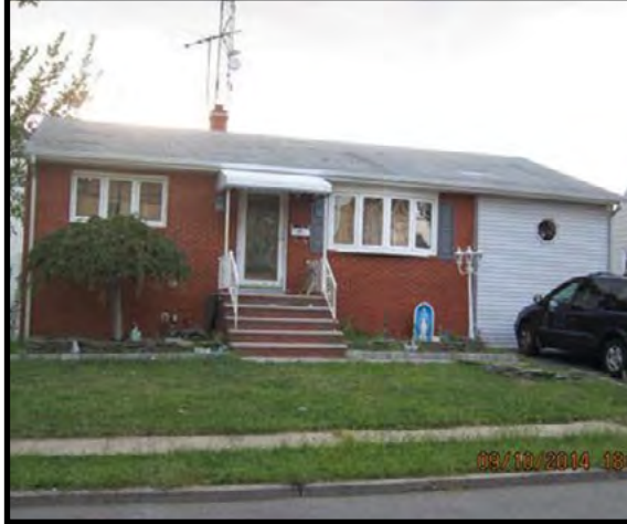
FORDS - Beautiful Ranch 2 bedroom contemporary stylish with many upgrades; kitchen cabinets will be replaced by different ones. it is being sold in AS IS condition. Buyer is resp. for Smoker cert and all repairs. $185,000
