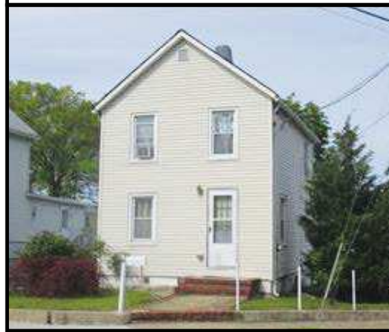
SOUTH RIVER - Very nice 2 bedrooms, hardwood floors, huge kitchen, formal dining room, very clean throughout, this property shows pride of ownership. $219,000
