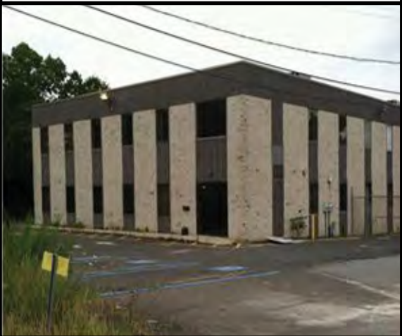
PERTH AMBOY - WHAT A DEAL!!! HIGH TRAFFIC LOC. MINS FROM NYC, NWK AIRPORT, MAJOR HWYS(TRNPK/PKWY/440/287/35/1&9/OUTERBRIDGE) BLDG CAN BE DIVIDED INTO 2-6000SQ FT UNITS OR 1ST FLR(4-750 SQ FT UNITS W/ A COMMON AREA). COULD BE USED FOR MULTIPLE BUSINESS/ATTORNEYS/CORPORATE OFFICES/DOCTORS/ADULT OR CHILD DAY CARES/HOUSE OF WORSHIP. BUILDING IS WAITING FOR YOU TO BRING YOUR DREAMS TO LIFE. $1,499,900
