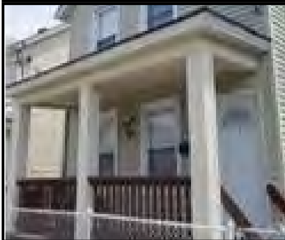
PERTH AMBOY - Central AC and roof are about 3 years old, living room, dining, private patio, granite counter top, new vanity, freshly painted. Close to school, all major transportation, food store, and more. $165,000
